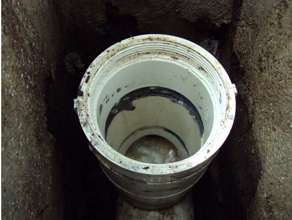
Figure 31. Standard T style PVC pipe that holds chlorination tablet holder
