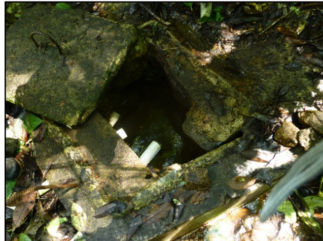
Figure 8: Spring Box with Lid Open
