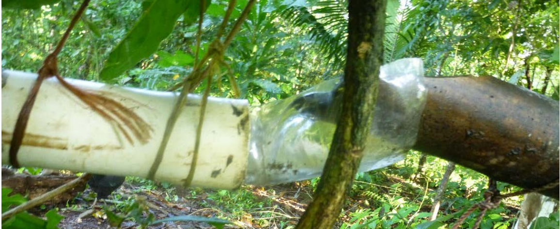
Figure 29. Sections of current pipe system in Quebrada Caracol community
