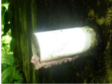
Figure 10: Termites entering water storage tank overflow pipe
